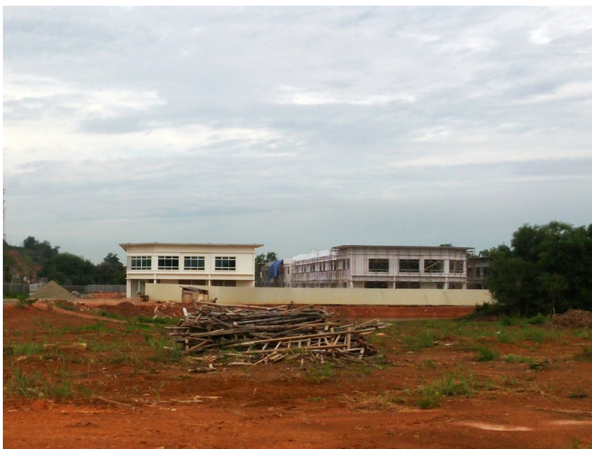
Figure 6: A township is being developed on an ex-mining land in Pengerang, Johor
