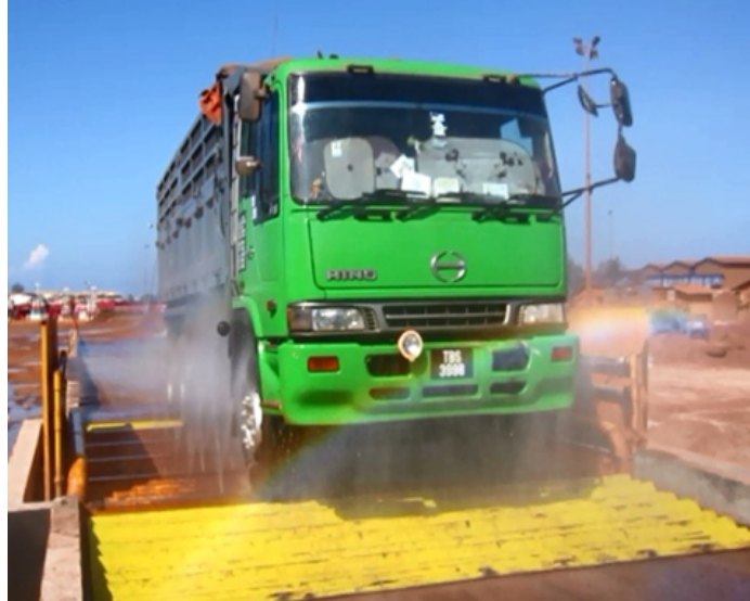
Figure 4: Wheeler Washer installed onsite
