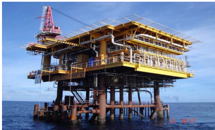
Figure 2.8-10 Typical wellhead platform in offshore Malaysia (Courtesy: Technip)
