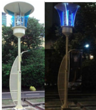
Figure 2.8-3 Installed wind-solar hybrid street lamp post with (ODGV) at Mid Valley, Kuala Lumpur
