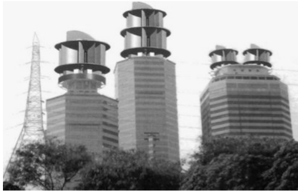
Figure 2.8-4 3-in-1 building integrated wind-solar hybrid energy system with rain water collection features retrofitted on top of some the buildings in Kuala Lumpur Malaysia (Source: Chong et al., 2011)
