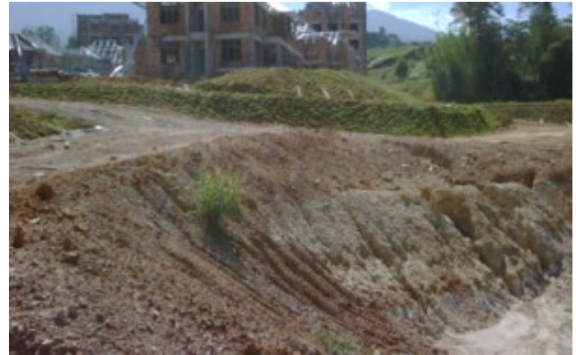
Figure 11: Spot turfing onto bare soil on a slope
