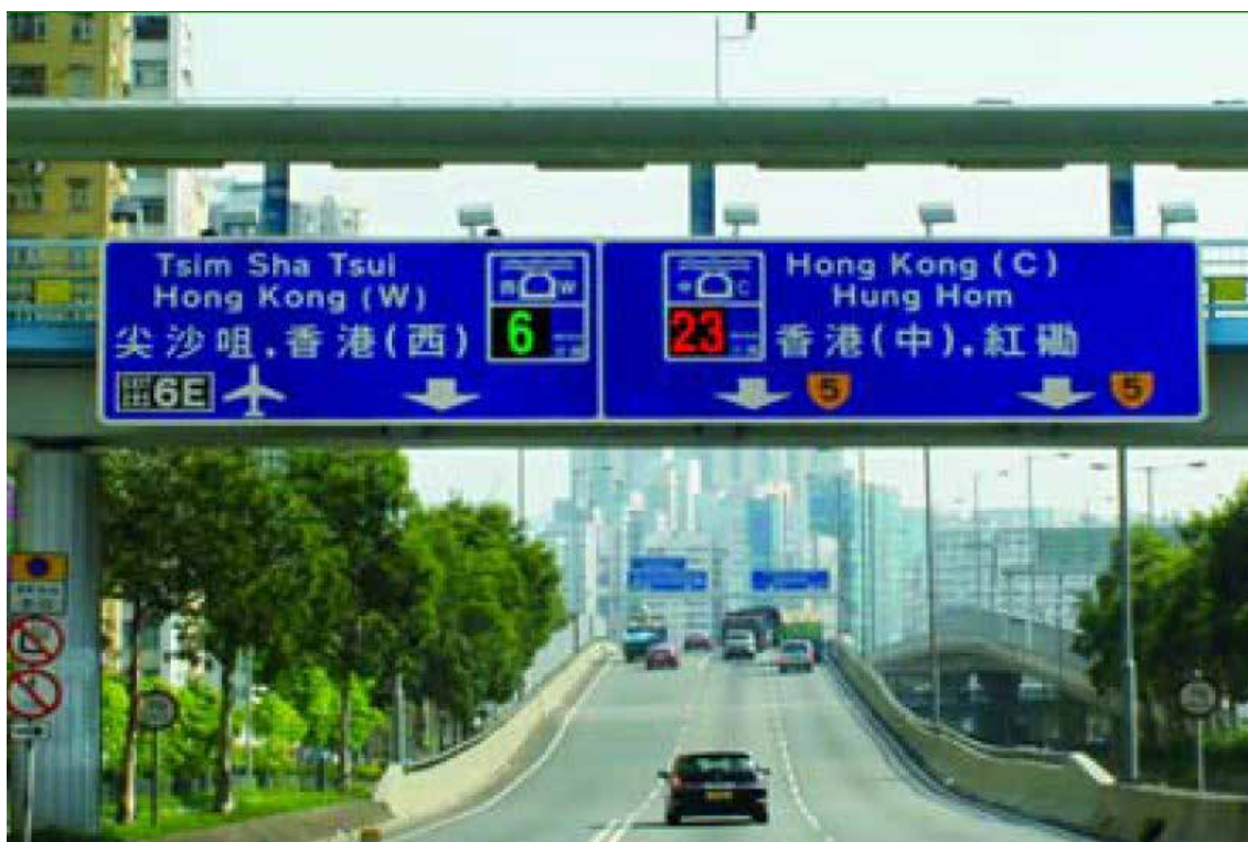
Figure 5.10 The Journey Time Indicator System LED time indicator in Hong Kong
