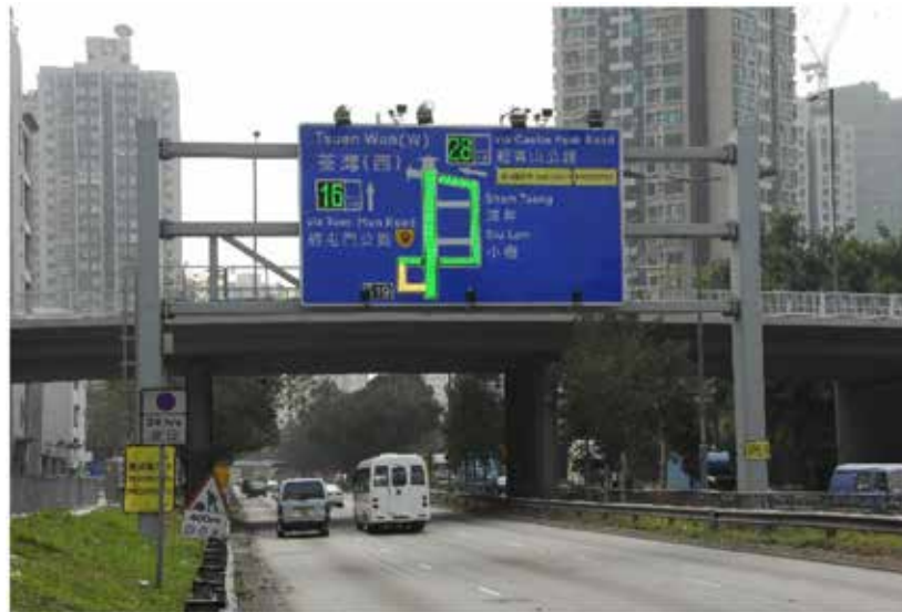
Figure 5.12 The Speed Map Panels in Hong Kong displays the schematic map of major routes ahead as well as the estimated journey time. The displays are colour-coded with green, amber and red to represent different traffic conditions: red represents congested traffic, amber represents slow traffic and green represents smooth traffic
