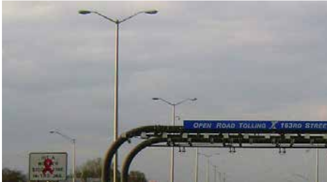
Figure 5.33 Open road tolling lane
