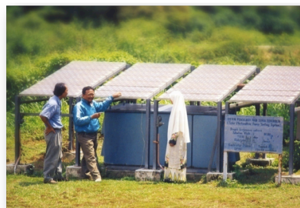
Figure 7.40 1.2 kWp water pumping system
