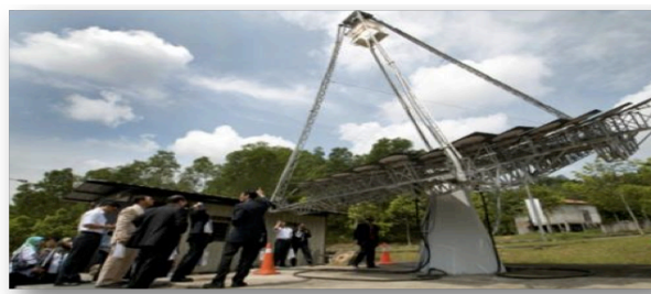
Figure 7.55 Grid-connected dense array concentrator PV system
