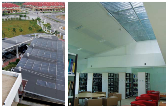
Figure 8.17 Among the energy-efficient measures (solar panels, natural lighting) of the net zero-energy office building of Pusat Tenaga Malaysia
