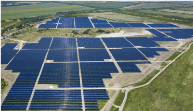
Figure 7.12 The 78 MW Phase 1 of the Senftenberg Solar Park in Germany generates power for 25,000 households
