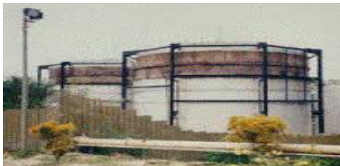
Figure 4.4 A floating roof closed-tank anaerobic digester system for POME biogas capture in Malaysia
