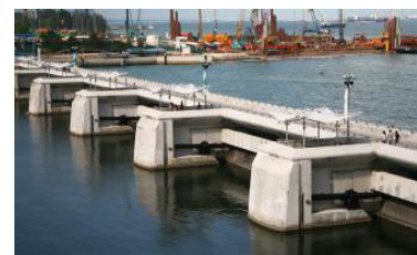
Photo 36: The Marina Barrage provided freshwater storage sourced from urban stormwater
