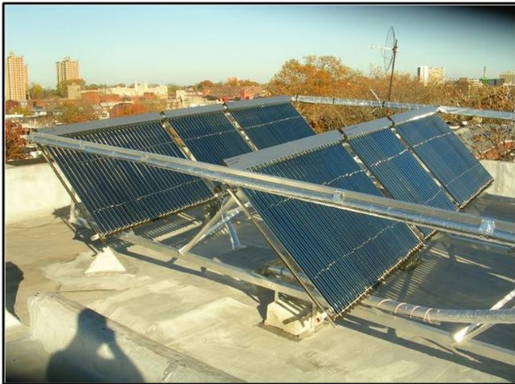
Figure 6.6: An Array of Evacuated-Tube Collectors on the Roof of a Commercial Building
