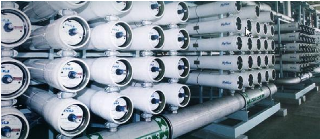
Figure 13: Membrane technology used in the production of NEWater
