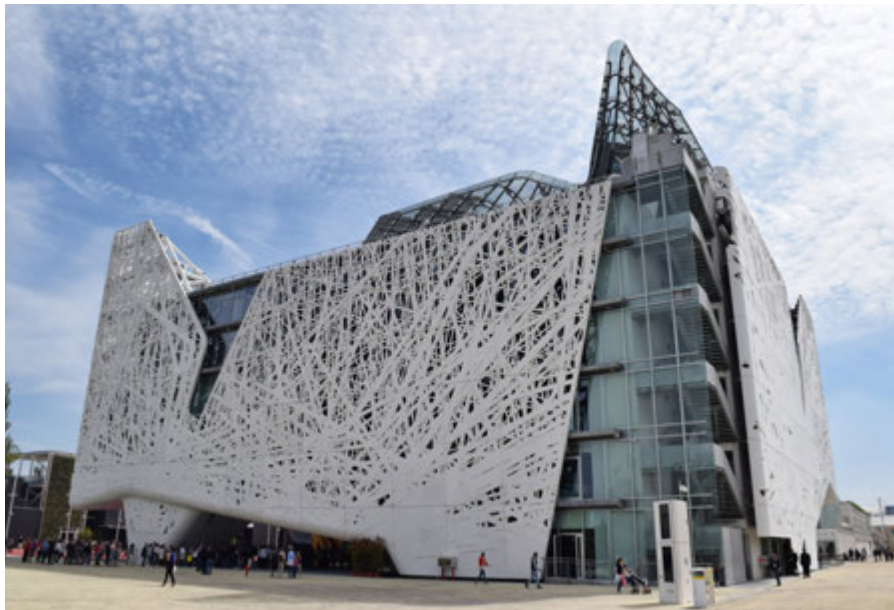
Palazzo Italia in Milan, Italy Italcementi (2020)
