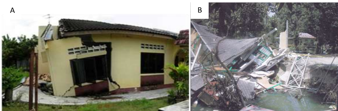
Figure 1. Sinkhole disaster has destroyed residential homes
