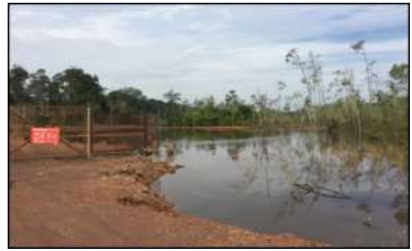
Figure 3. Flooding and overflow at Sungai Jemberau on 2 February 2017
