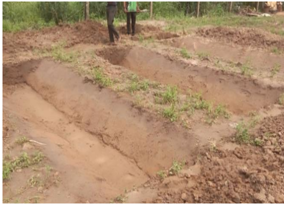
Figure 1. Construction of trapezoidal channels in Agricultural and Bio-resources Engineering experimental site
